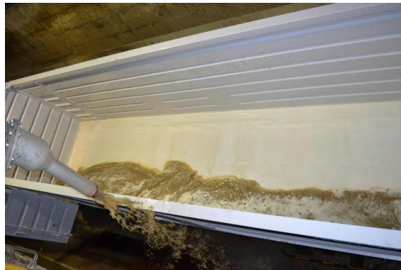
Figure 207: Type L, Washing out of bulk cargo B.2.3.3.
