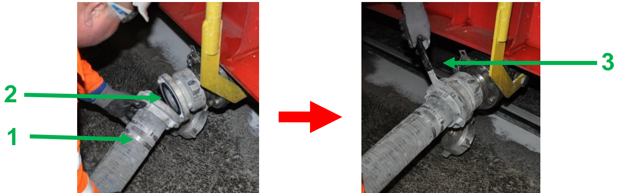
Figure 153: Type G, Before emptying D.1.2.
